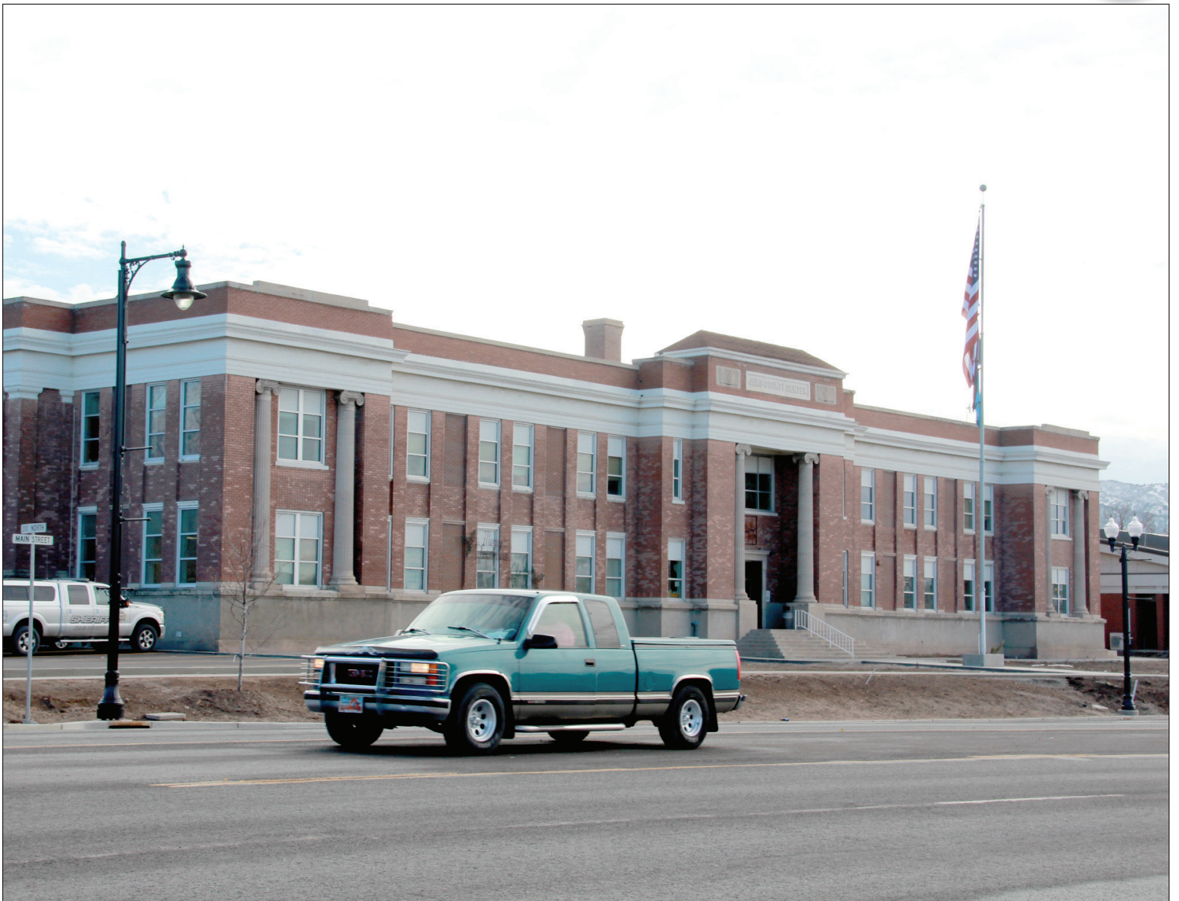
REMODELING TO START IN JANUARY • Areas of the Juab County Building will be remodeled in January according to the Juab County Commission. The Clerk’s office and the south stairs are areas slated for work. Ryan Lynn Construction was awarded the contract.
