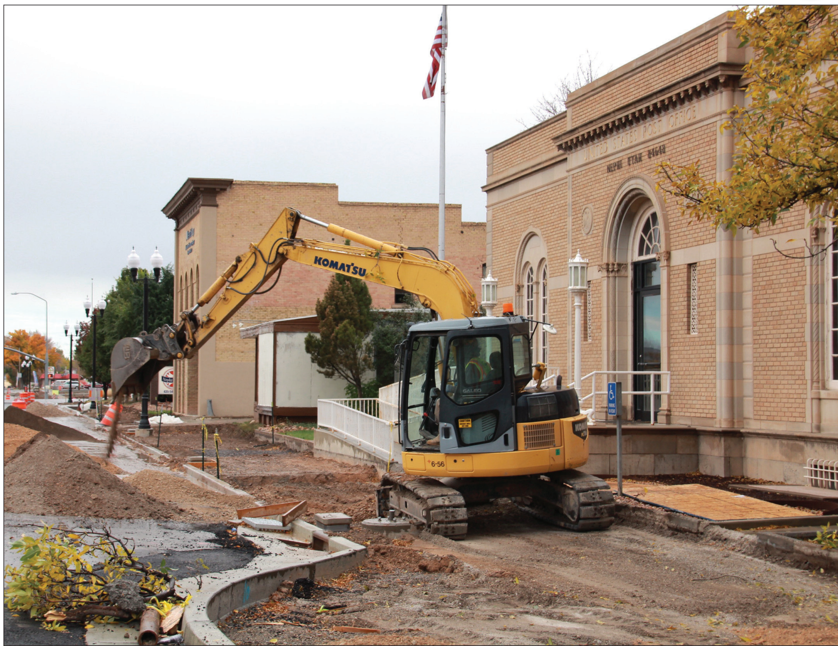
ALMOST TO THE END • UDOT crews were out working in the rain on Monday morning trying to keep the Main Street project on schedule. In the past week they installed the new light poles along Main Street. The consensus says they are beautiful. UDOT update on page 2
