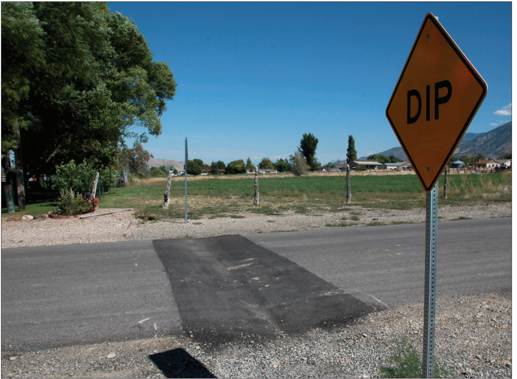
DIP CAUSING CALLS TO MONA OFFICIALS • This dip in the road at 300 West and 300 South in Mona has a few residents protesting to city council members. Katrina Long, council member, wants the dip to be reversed or modified.
