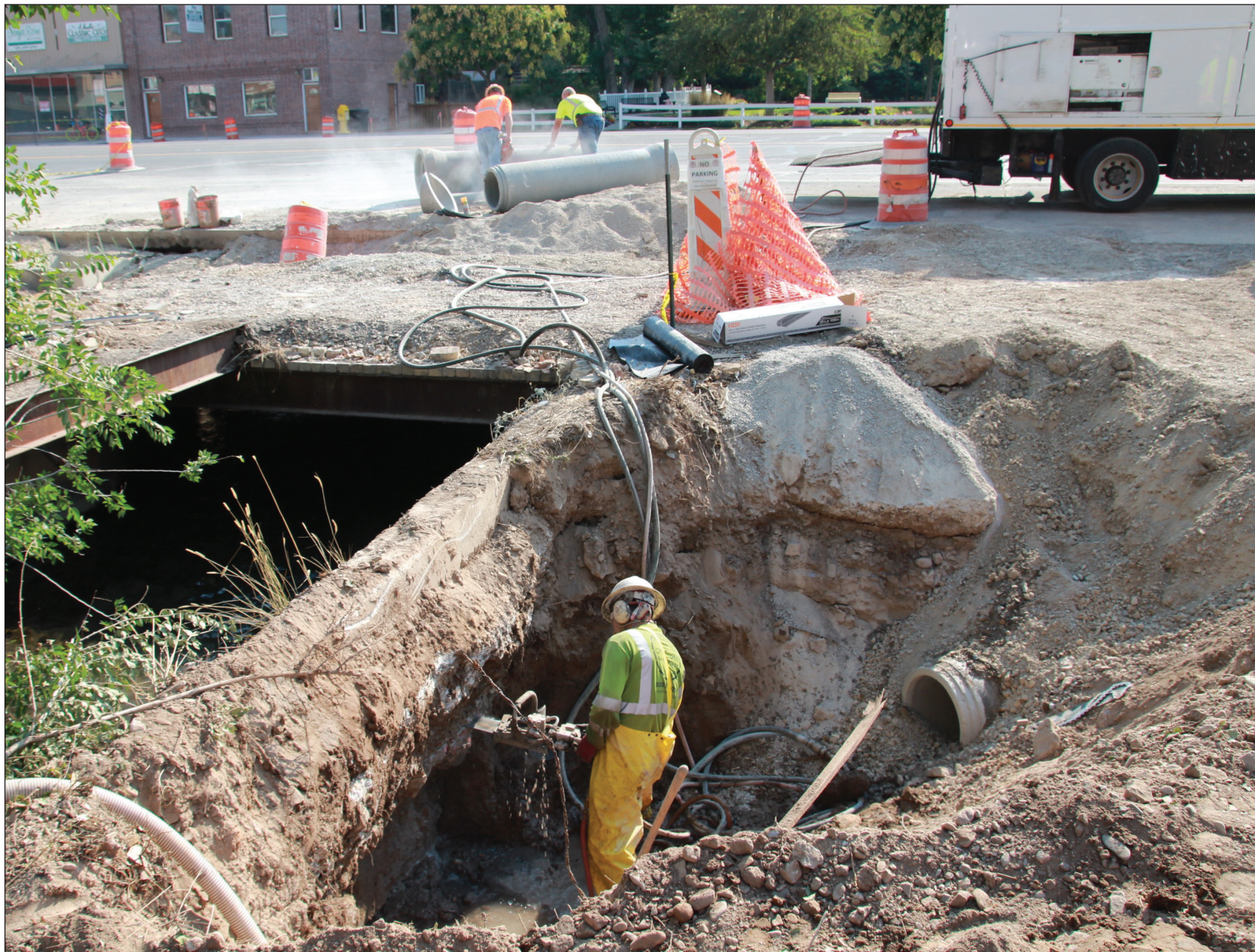
MAIN STREET WORK CONTINUES • Crews continue to work on the Main Street Project. Above, worker cuts through the wall on the south side of Salt Creek so that drainage pipes will be able to drain into the creek. Crews have been finding buried tanks and basements that were long forgotten.
