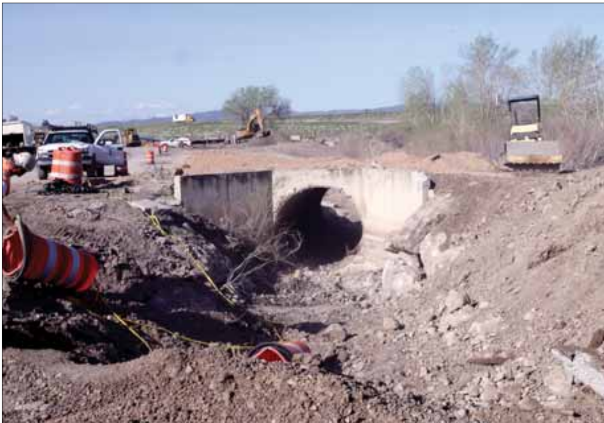
COMING RIGHT ALONG • The East Juab Water Efficiency Project, a joint project of Central Utah Water Conservancy District and Nephi Irrigation Company, is progressing at the mouth of Salt Creek Canyon. 2,200-feet of pipeline us being installed to lessen the amount of water being lost to seepage at this point.
