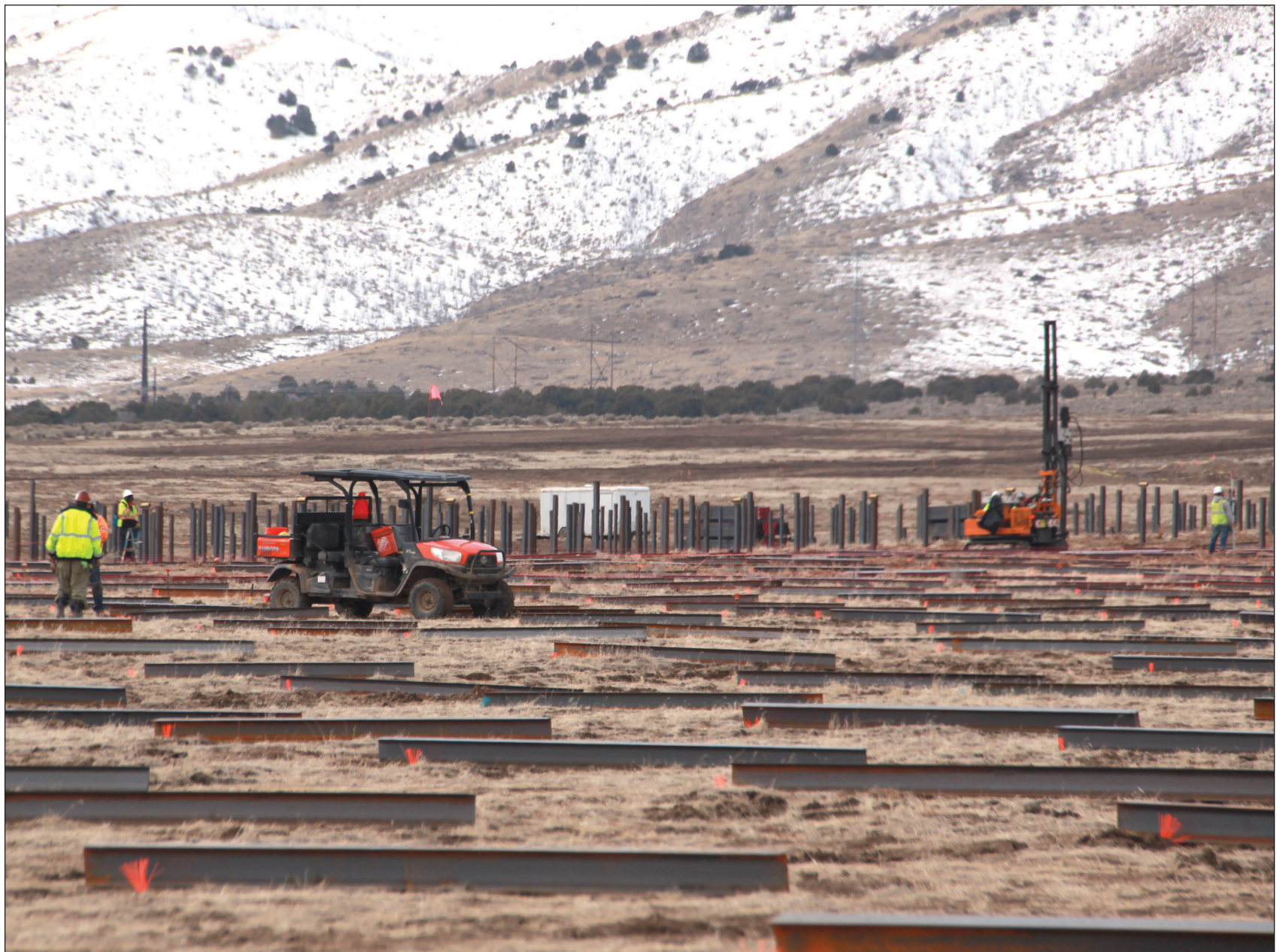
CONSTRUCTION STARTS • Clover Creek Solar is beginning construction west and north of Mona. The project should take between 6-9 months to complete. Above, crews are using a pile driver to install support posts for the panels.
